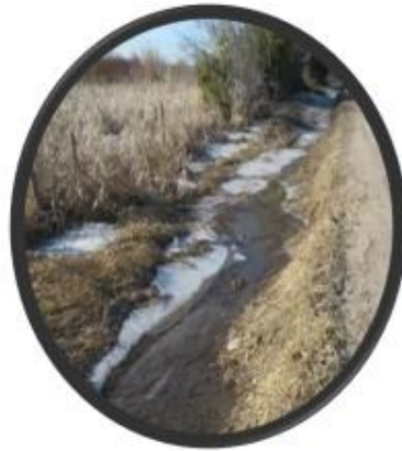
D) Drainage Ditch
