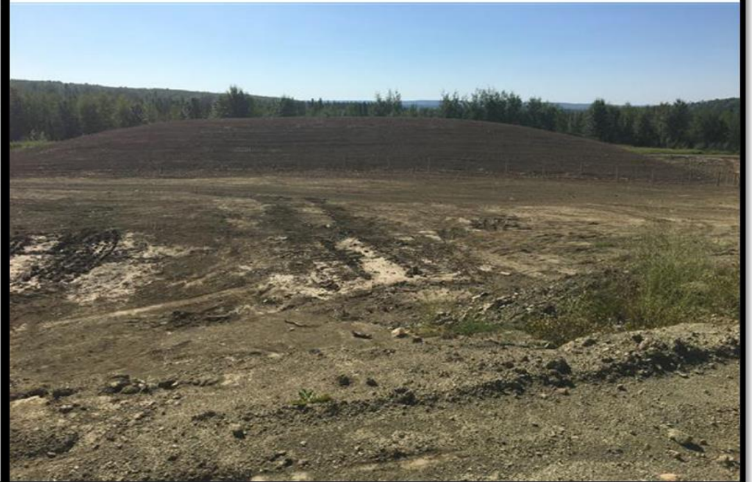
AUGUST 18, 2020 FINAL INSPECTION
