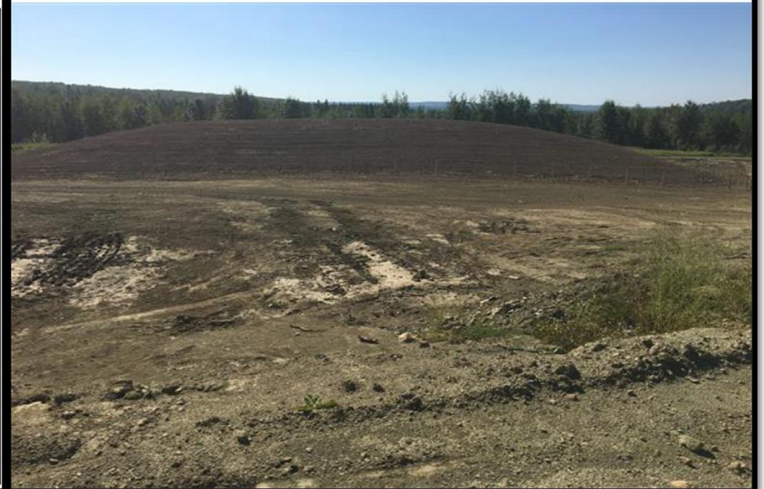
AUGUST 18, 2020 FINAL INSPECTION
