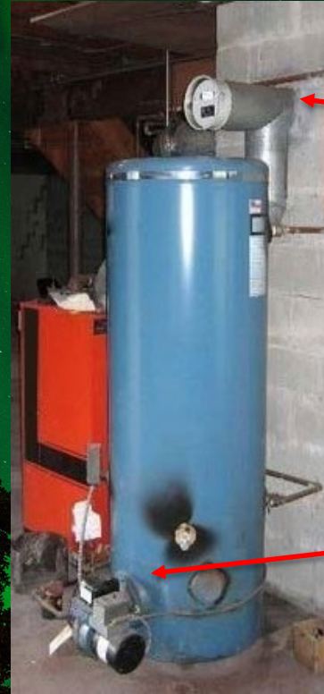
Diesel hot water tank
