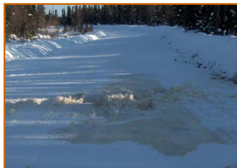
Image 4: The presence of water and slush damages the winter road making travel difficult.
